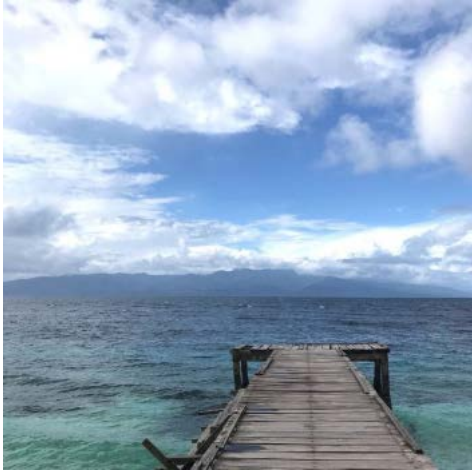
The old WW2 jetty at Liang airfield
