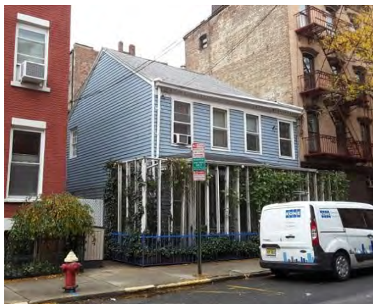
206 Third Street (Property ID -1199299686), built ca. 1850, is one of the earliest surviving wood frame dwellings in the Hoboken Historic District as well as one of few examples of the Greek Revival style, featuring a denticulated cornice; full façade front porch with columns; and an original or early door surround with sidelights and multi-light transom.
