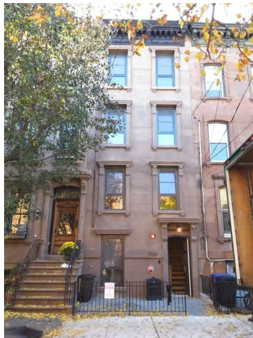
920 Bloomfield Street (Property ID 721301392). Here the basement was eliminated and the floors re-aligned with the first floor above DFE (slightly above sidewalk grade). While this property was still recommended as contributing due to the retained height, massing, upper floor openings, and cornice, its overall integrity is diminished and the streetscape has been adversely affected.
