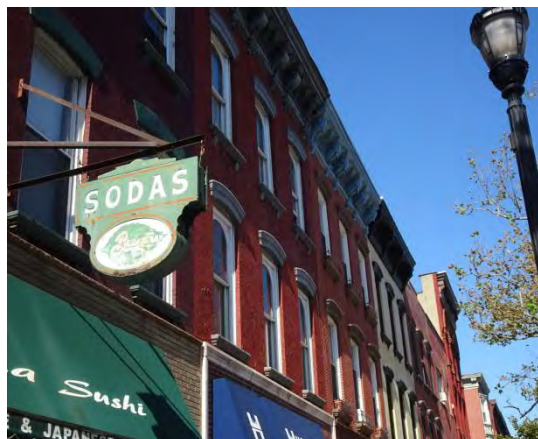
Typical mixed-use, Italianate-style rowhouses along Washington Street.
