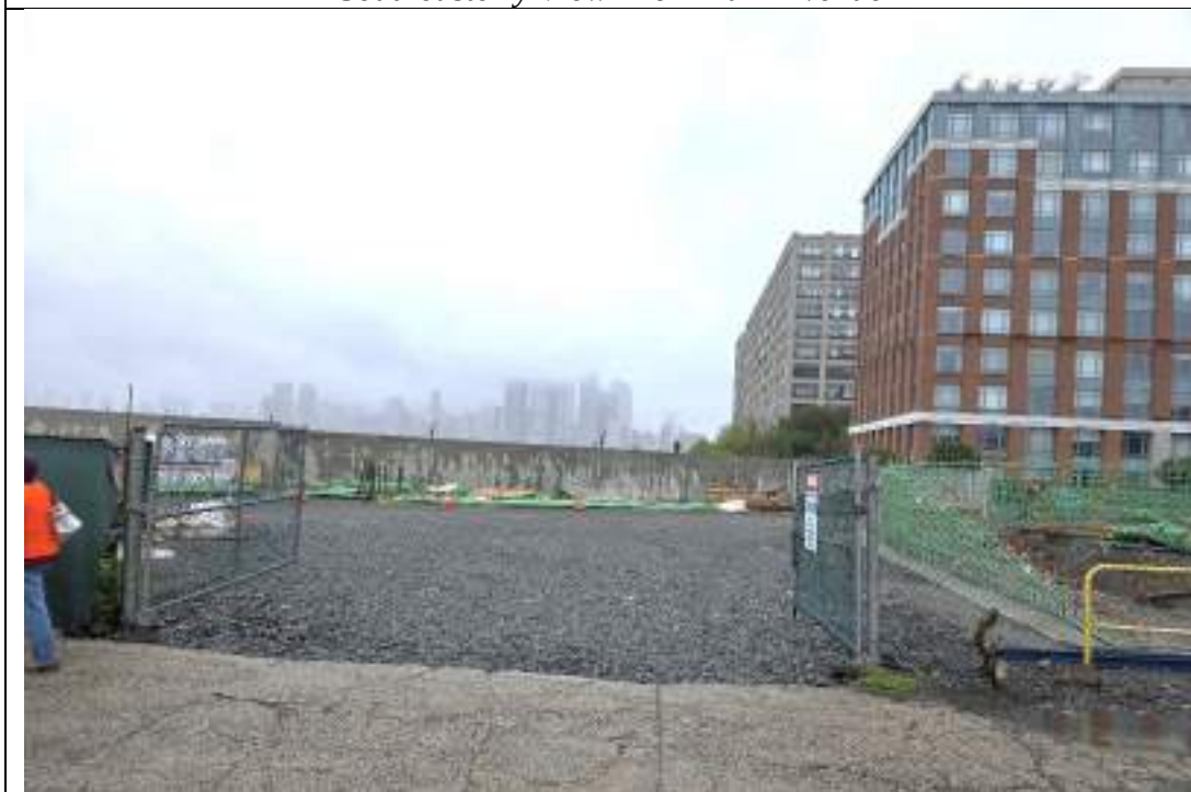
Easterly View From Park Avenue
