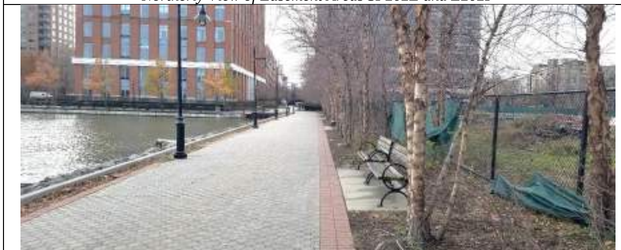
Southerly View of Easement Area SP202E
