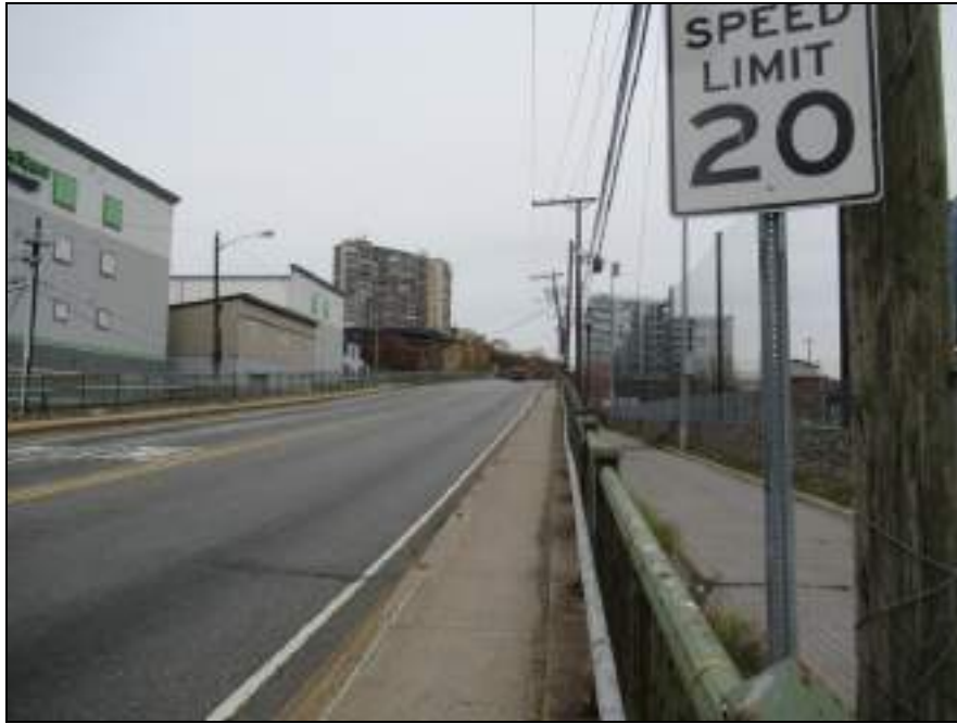
Northerly View along Willow Avenue (Taken November 2023)
