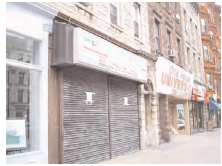
Solid security gates should be prohibited.
