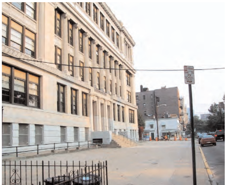
The historic Demarest School, which was recently renovated, is home to a middle school and a charter school. If vacated, it should house public uses such as an arts facility or additional charter schools.
