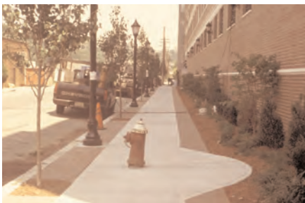
Pedestrian-friendly design involves paying more attention to details. Leaving this hydrant in its original location blocked the sidewalk and cut into green space along a newly constructed building.
