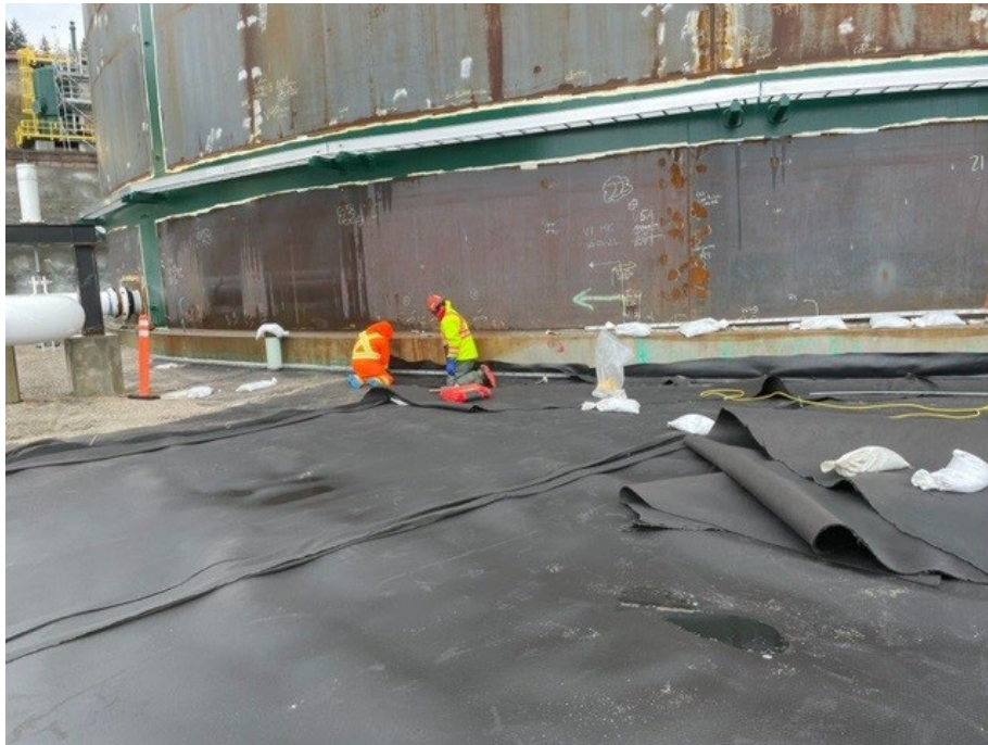
Mechanical connection of 40 mil liner to outside tank ring beam on 6" centers
