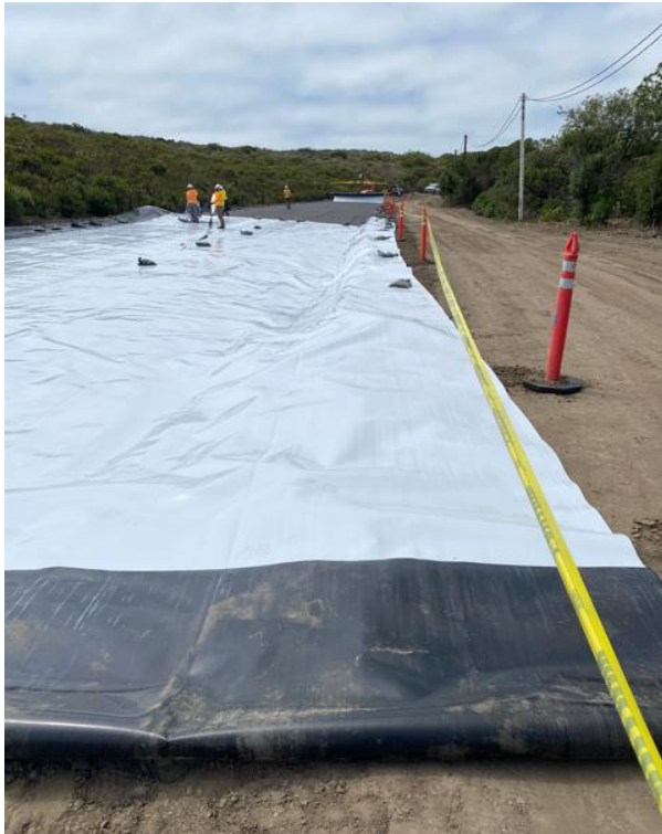
First layer of 40-Mil Blended LLDPE/HDPE
