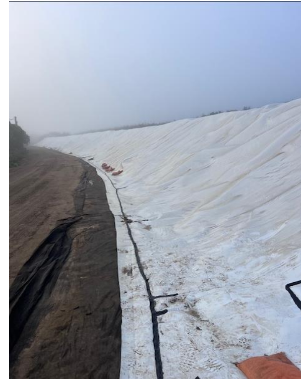
Capping Blended LL/HD liner welded to base liner
