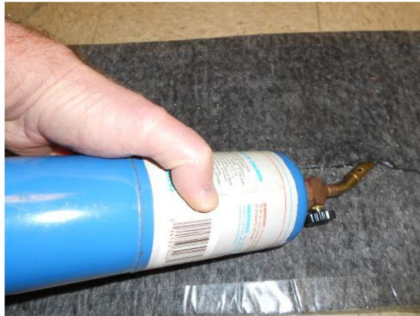
(a) Propane torch seaming GCL
