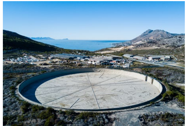
Figure 4. Installed 45 mil R-PP potable water tank liner floating cover, South Africa
