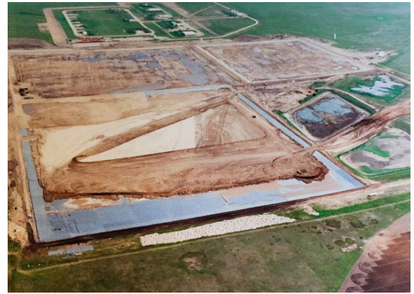
Figure 2. PVC geomembrane lined municipal effluent pond
