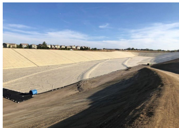
Figure 9. R-PP liner installed for large raw water storage pond in Colorado, USA
