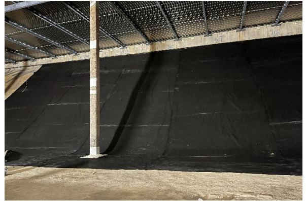
Figure 5. Geomembrane relining of underground concrete reservoir in Arizona
