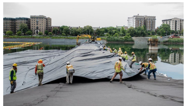
Figure 5. Installation of R-EIA geomembrane for a water reservoir in Maryland, USA
