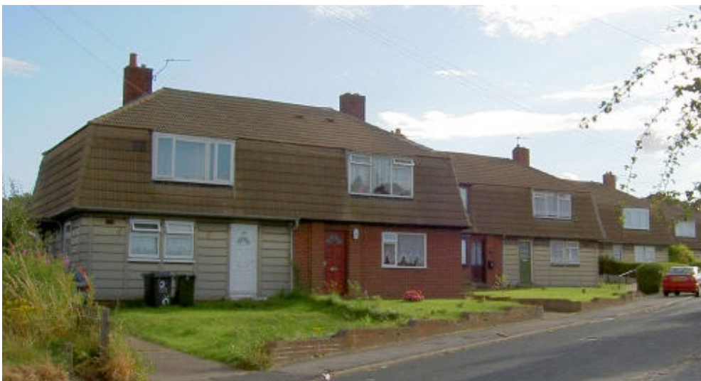
Contemporary photograph: semidetached houses with distinctive mansard roofs in Darfield, South Yorkshire, © Steve Fareham
