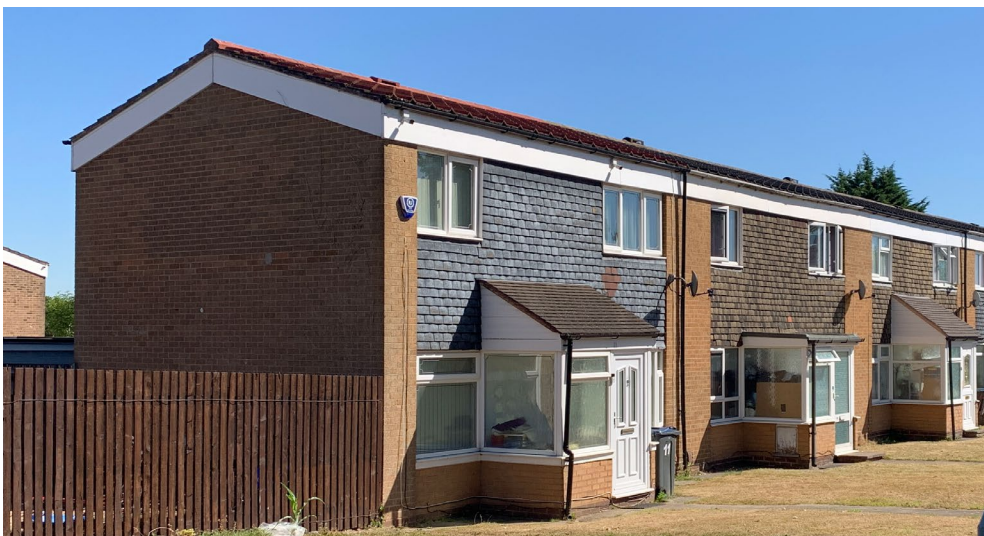
Example project: Birmingham City Council terraced Bryant Low Rise cross wall houses in Birmingham before retrofit
