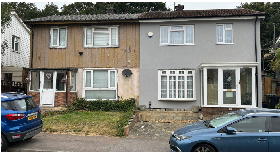
Contemporary photograph: BISF semidetached houses in London Borough of Redbridge; the lefthand semi is in original condition apart from newer porch, doors and windows
