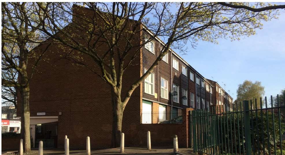
Example project: Nottingham City Council's terraced cross wall houses in Nottingham before retrofit, the houses are next to flats and bungalows of similar construction
