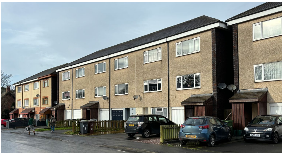
Example project: Wolverhampton Homes' four-bedroom terraced Wimpey No-fines houses in Wolverhampton before retrofit (a previous retrofit has been undertaken)
