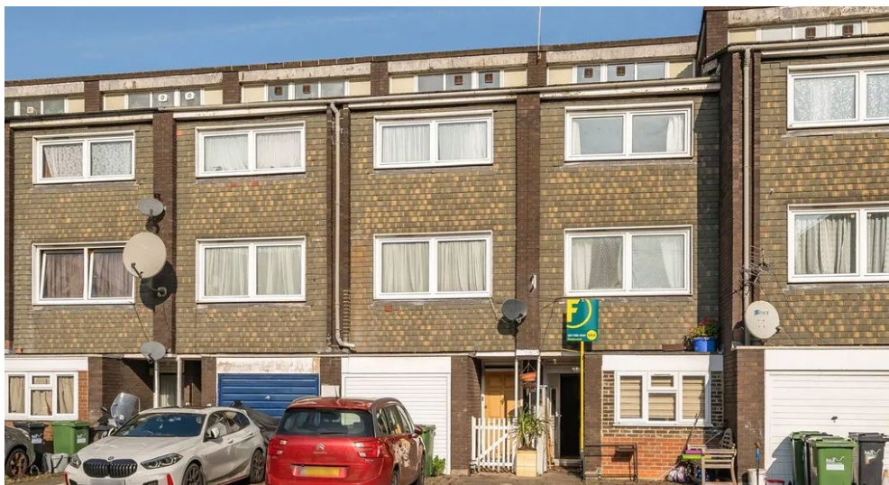
Example project: Hammersmith & Fulham Council's terraced houses in Fulham before retrofit
