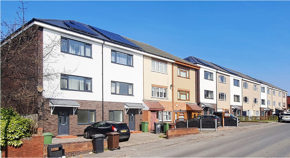
Example project: four-bedroom terraced Wimpey No-fines houses in Wolverhampton after retrofit for Wolverhampton Homes (10 homes were upgraded)
