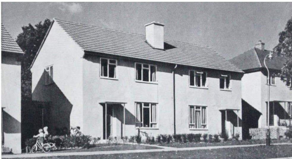
Historic photograph from George Wimpey & Co. Ltd. publication: two-bedroom semidetached Wimpey No-fines house type built at Farnborough, Hampshire
