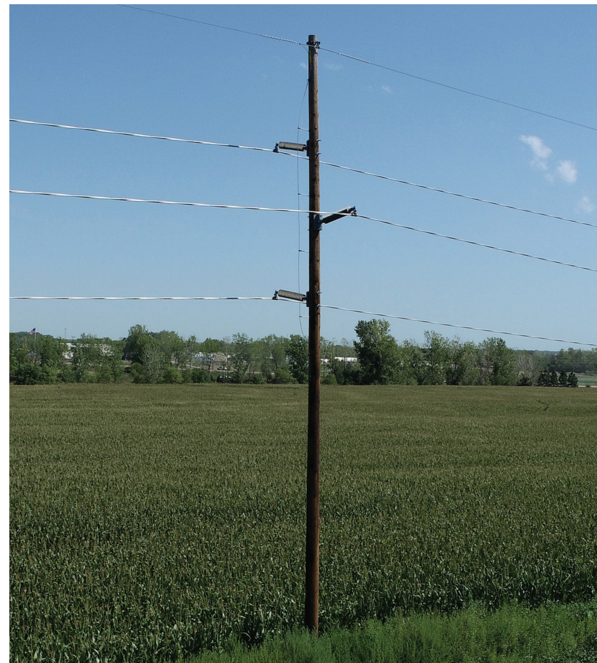
TYPICAL SINGLE-POLE WOOD OR STEEL STRUCTURE
