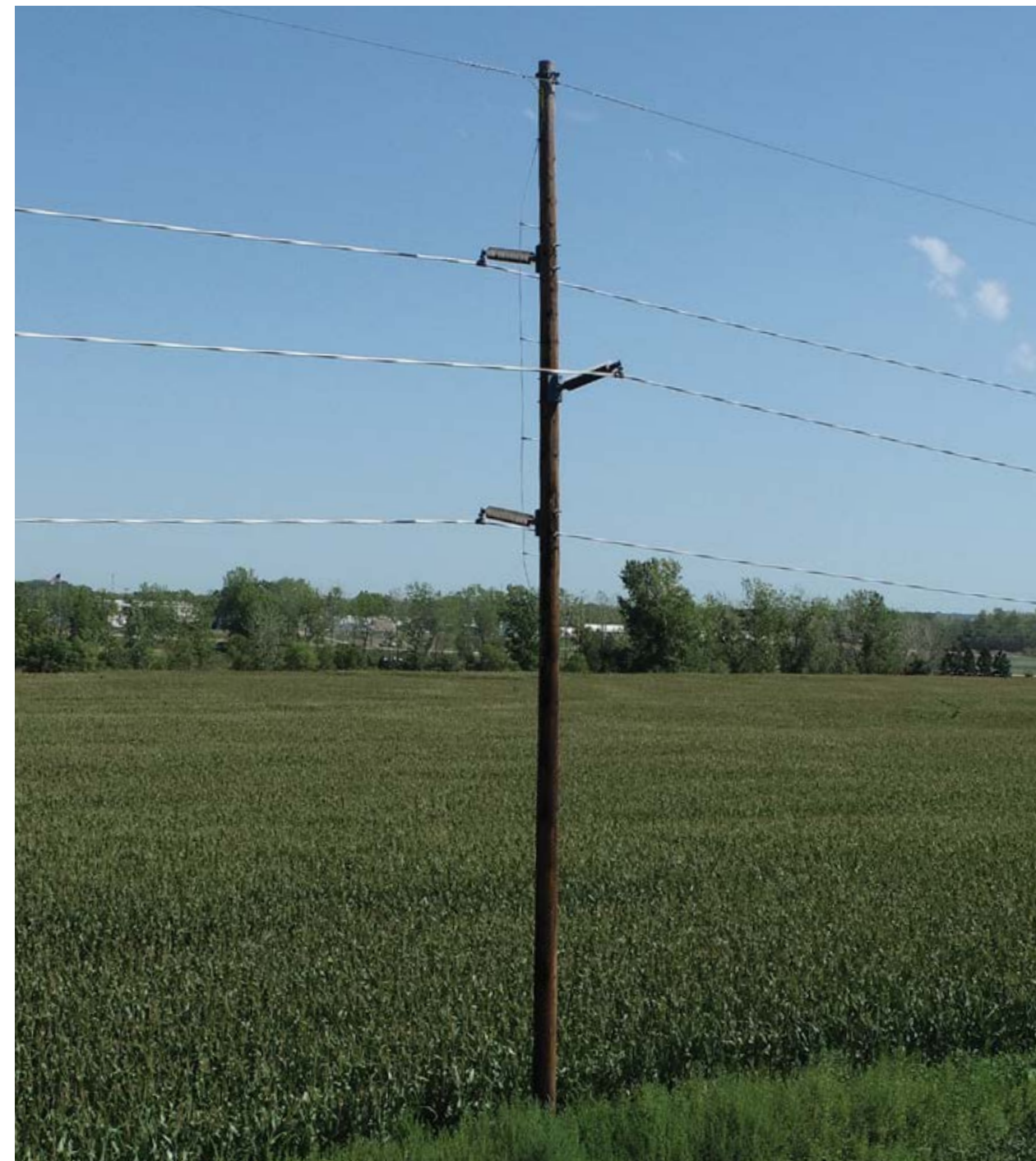
TYPICAL SINGLE-POLE WOOD OR STEEL STRUCTURE
