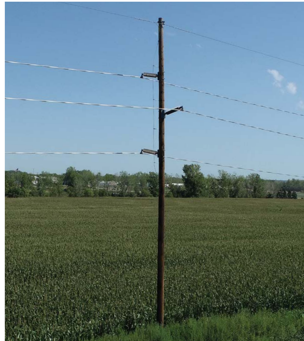
TYPICAL SINGLE-POLE WOOD OR STEEL STRUCTURE
