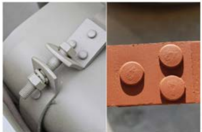
The two-part straps were held together with a bolt, almost like a ratchet. The rivets on these straps made by Ford had F script marks.
