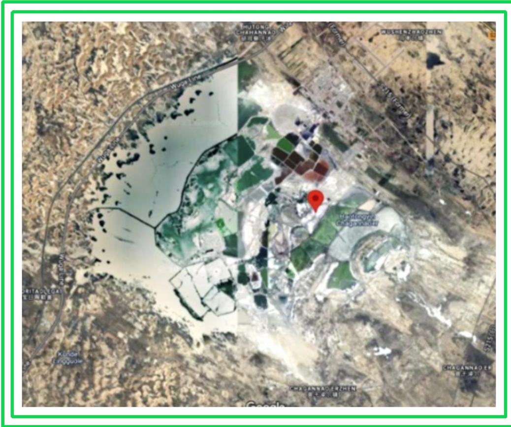
Solvent Extraction Facility Inner Mongolia, China
