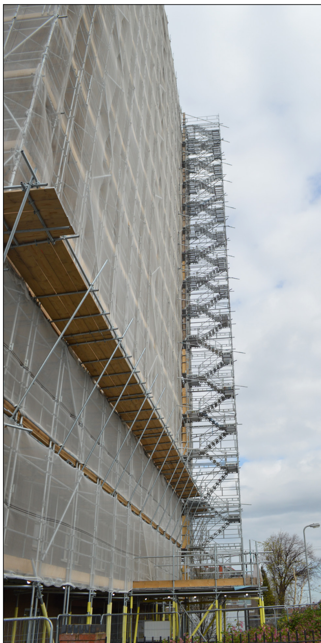
Figure 7 Where sheeted scaffolds form part of the escape route, do not sheet the stairways or ladder points so that smoke can escape and the fire and rescue service can gain access
