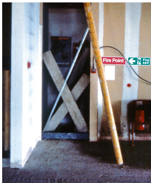
Figure 9 Avoid creating dead ends and misleading fire exit signage
