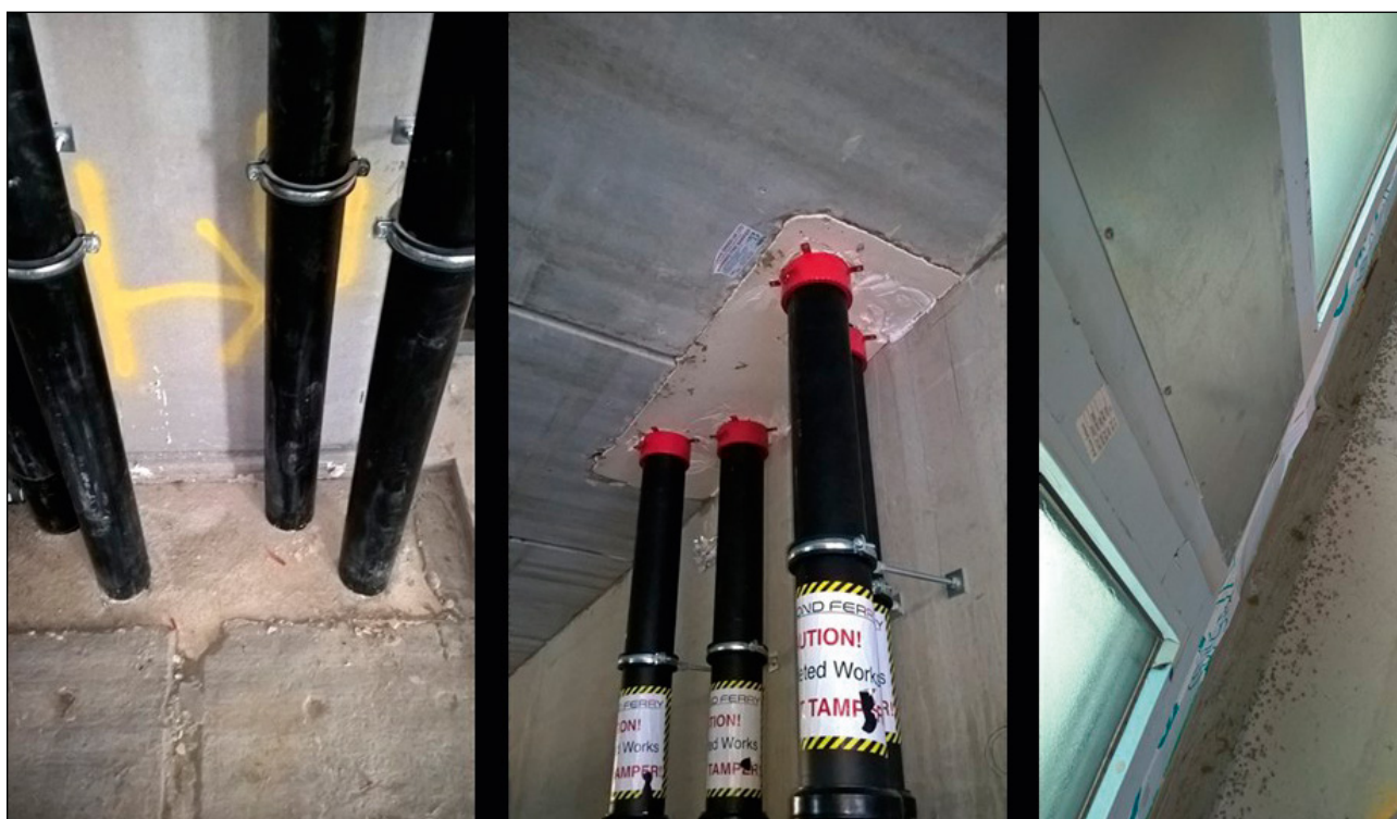
Figure 15 Fire stopping installed around penetrations made for services and in the gap around windows
