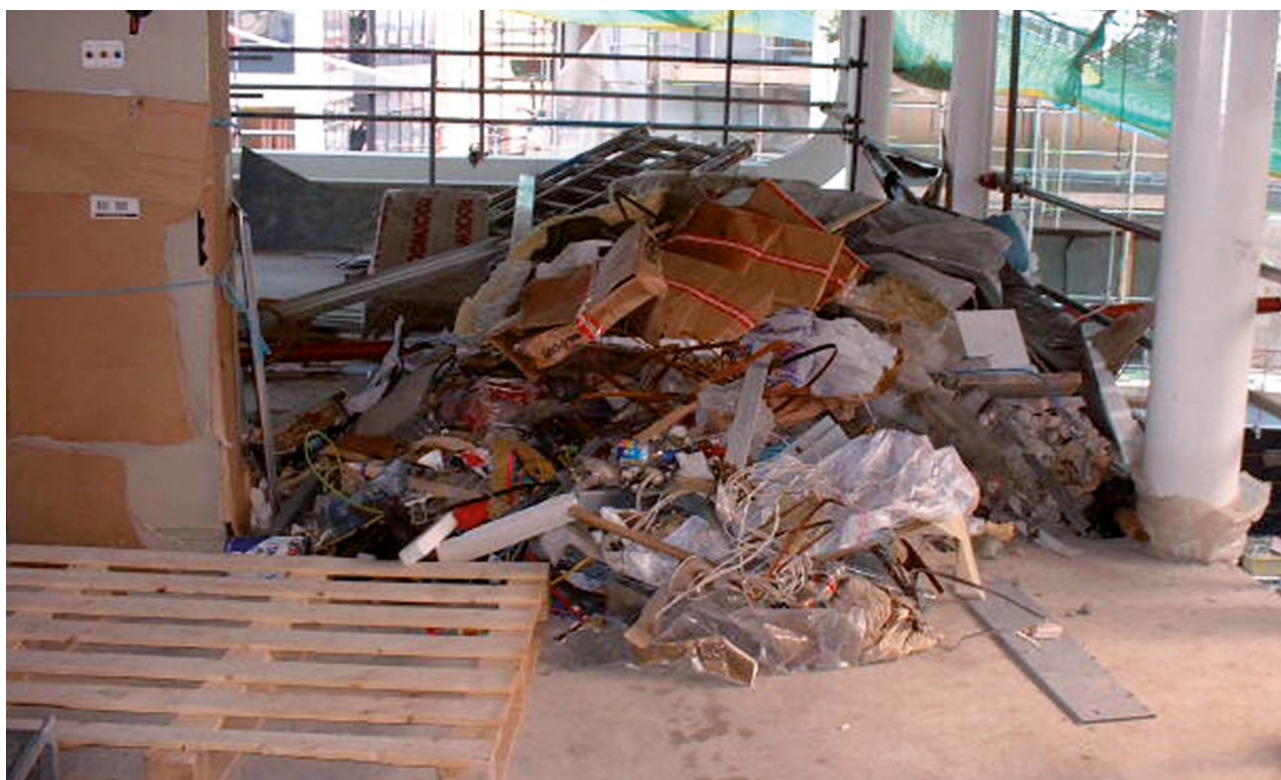
Figure 8 Most construction rubbish can burn. Make sure that it is cleared up and removed from the site as soon as possible
