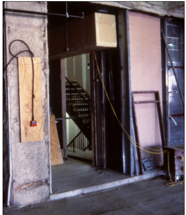
Figure 13b This escape route will quickly fill with smoke in a fire because no fire door is fitted
