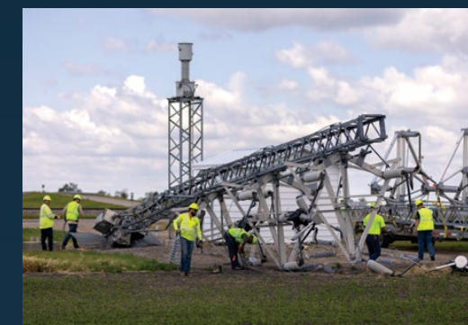
The Elm River line switch was one of the larger pieces of infrastructure destroyed by the storm's derecho winds north of Grandin. Its repair took collaboration between many power delivery teams.
