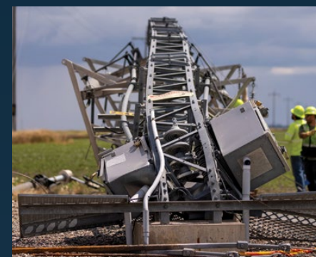
The Elm River line switch was one of the larger pieces of infrastructure destroyed by the storm's derecho winds north of Grandin. Its repair took collaboration between many power delivery teams.
