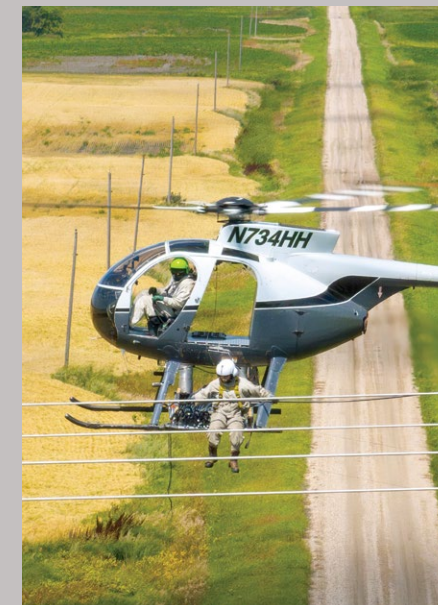
Airflow spoilers were added by hand while the line was still energized.
