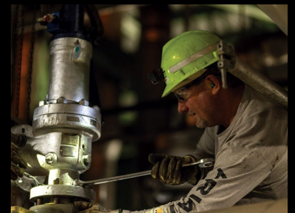
Minnkota Plant Mechanic Michael Grinsteiner installs a pressure relief valve on a feedwater heater.
