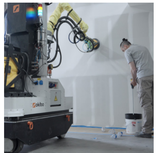
On display at the Summit: The Okibo robot performing autonomous drywall finishing in a live project simulation.
