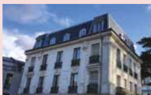
IBN's historic building with new roof
