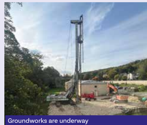
Groundworks are underway
