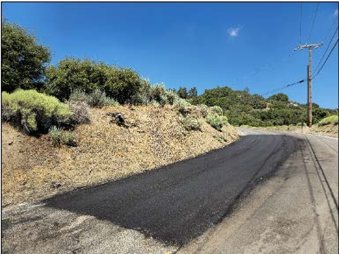
Overlay paving performed on Skyline Drive
