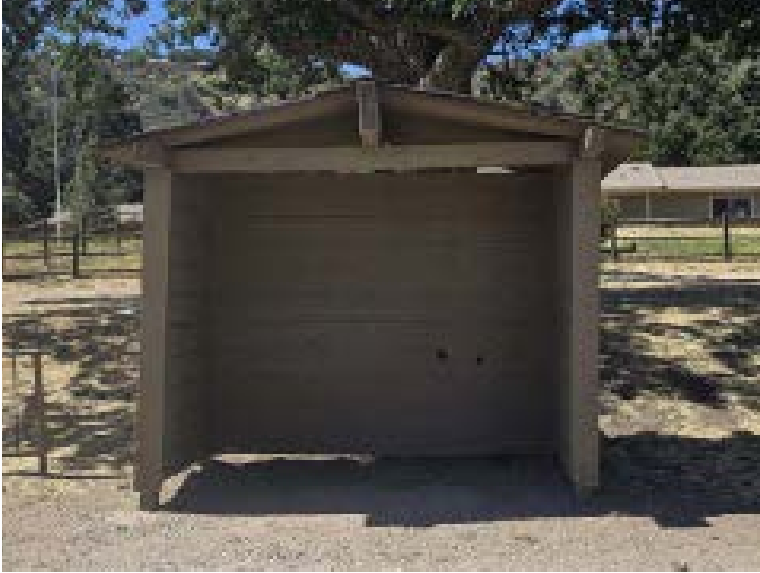
Condition of bus stop before work
