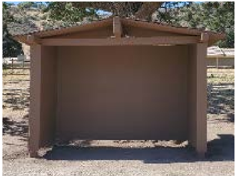
A little more dirt work needed and it will be ready for school to start!
