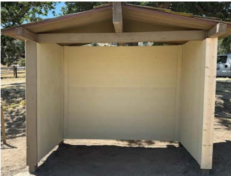
New siding installed
