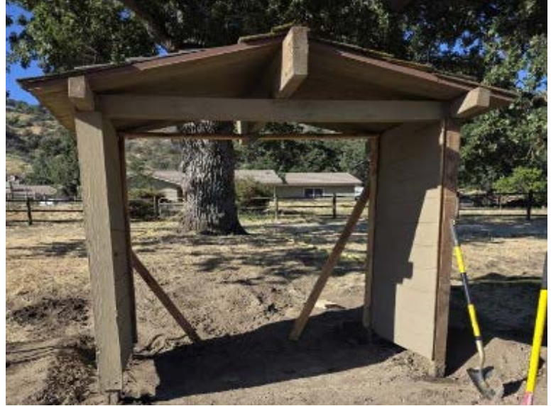
Back wall removed and one leg replaced
