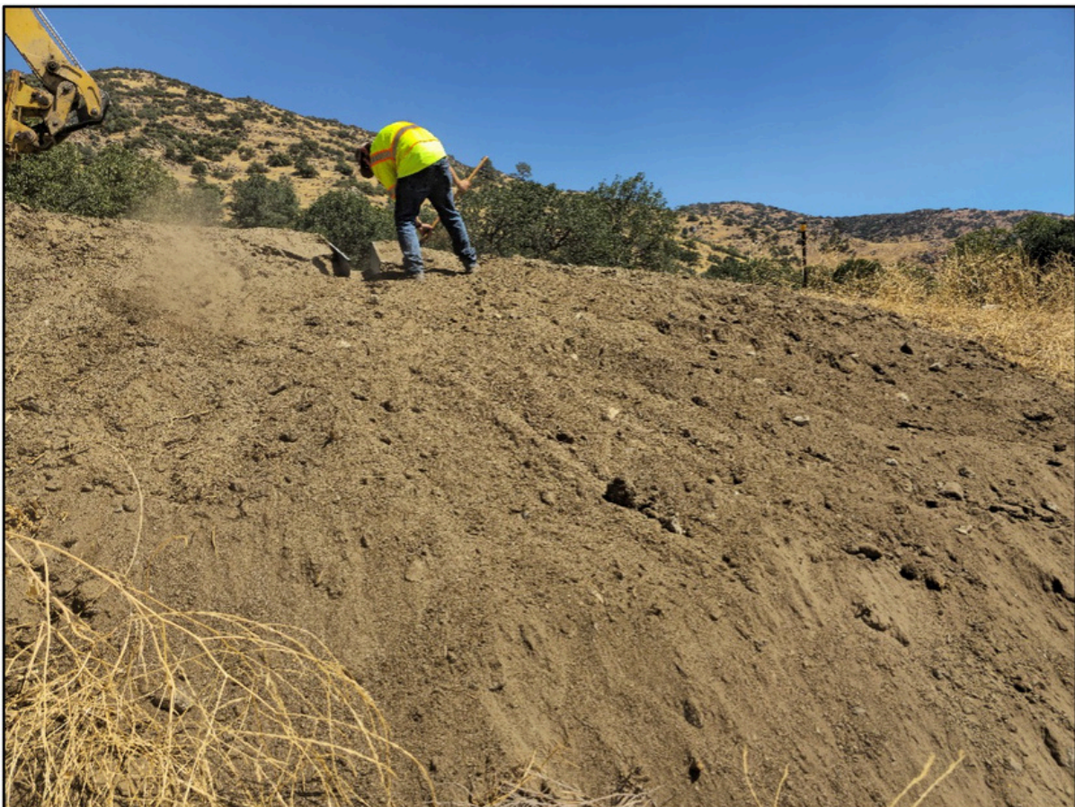
Erosion repair performed on 9/5, Bear Valley Rd.
