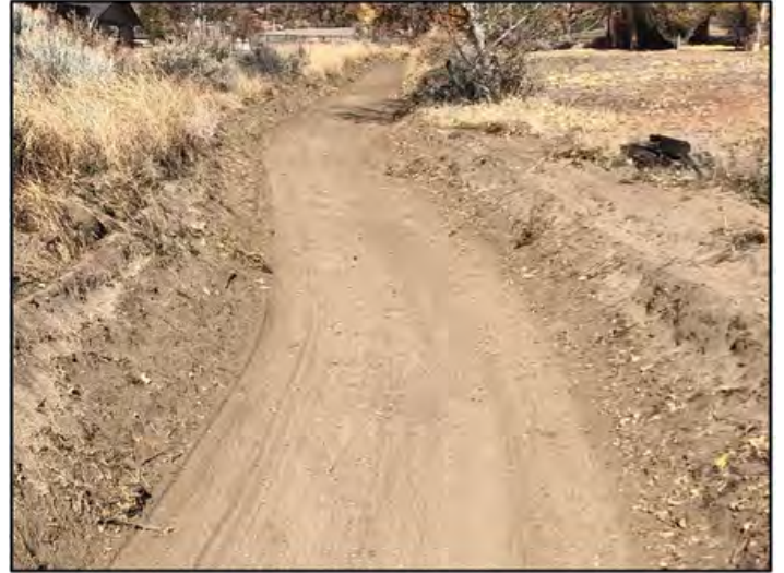
Drainage maintenance on easement at equestrian center
