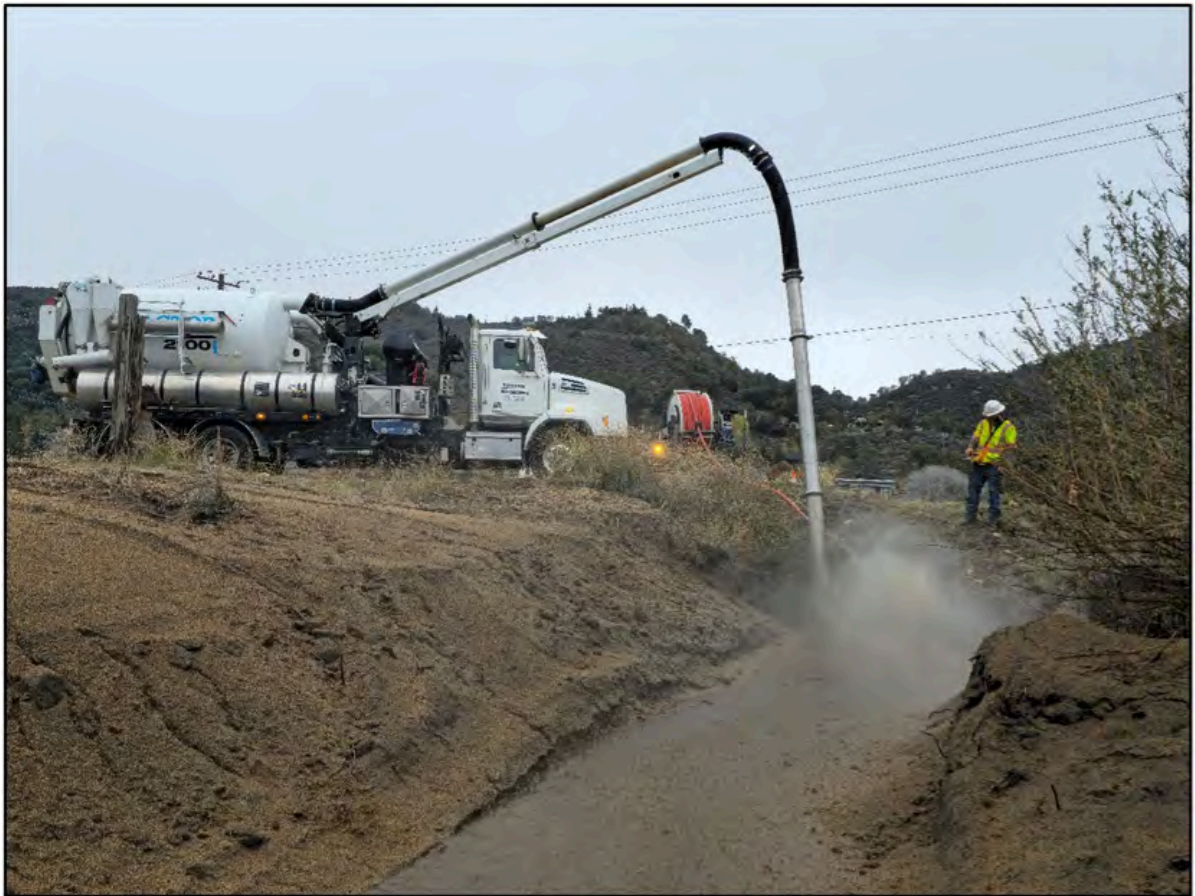
Hydro excavation being performed on Lower Valley Rd. (11/20)
