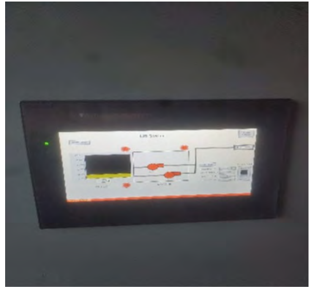
Lift Station PLC
