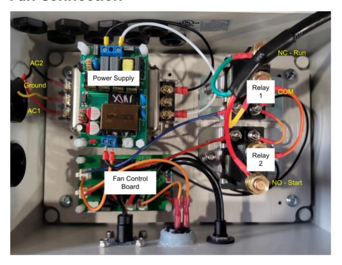
Connect the red AC1, black AC2, and yellow GROUND power wires to the fan power supply. Connect the yellow COM, red NO, and green NC relay wires to the switches. Refer to the common fan diagrams below for guidance on wiring connections. We strongly recommend emailing a picture and diagram of your fan to technical@grainanalyzers.ca for consultation on how to properly connect the fan control board.
