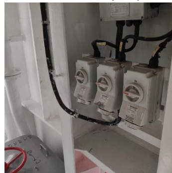
220V PS behind buoyancy-room
