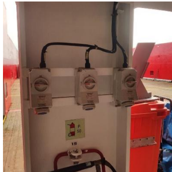
220V PS behind buoyancy-room
