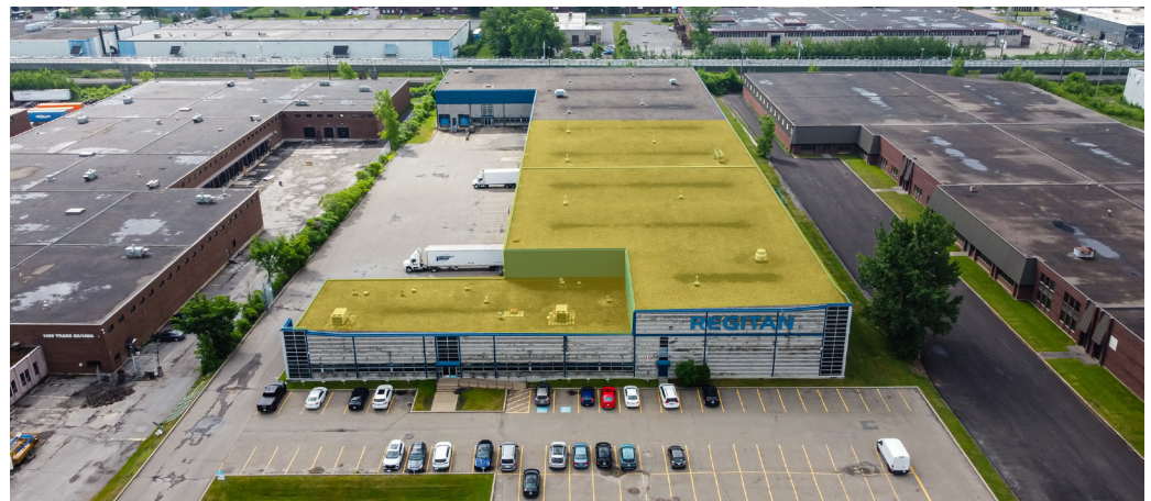
16 quais de chargements | truck-level doors
