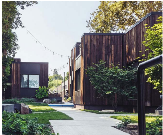
Walkway between two buildings in Spokane, WA. Photo credit: Jaydn Scandora/Unsplash
