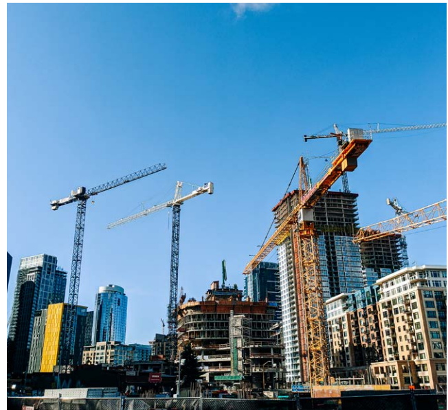
Downtown Seattle, WA construction cranes. Photo credit: Steve Banfield
