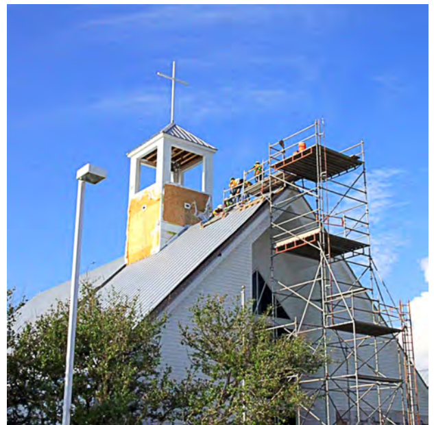
Finishing the bell tower
