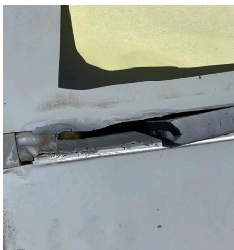
Figure 9 – Cohesive failure of sealant #2 in aluminum joint. Picture taken April 15, 2024.
