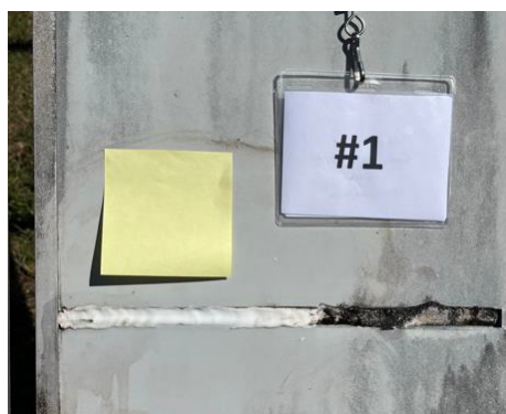
Figure 5 – Sealant #1 surface condition after cursory clean. Picture taken April 15, 2024.
