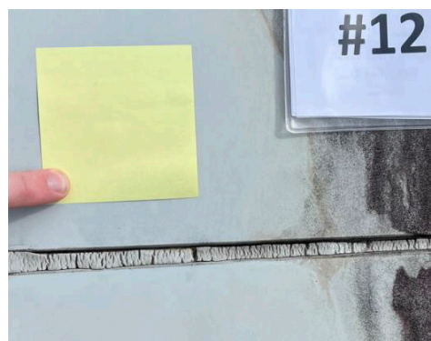
Figure 6 – Significant surface irregularities on sealant #12. Picture taken April 16, 2024.
