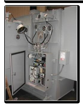
site. Note that the wiring from the various gauges is exposed SO cable. Entrances to the terminal box are made via watertight connections. The terminal box enclosure itself provides a <u>degree</u> of protection against:
