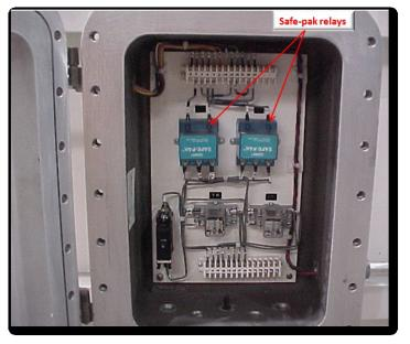
Adjacent is a close up photo of the previous image detailing the control enclosure. The enclosure serves as a centralized point in which to terminate the output from a variety of gauges and devices located on the transformer including liquid level gauge, thermometer, pressure vacuum gauge, and sudden rise pressure relay. The outputs from these devices control the operation of connected equipment, largely through relays. To prevent the
