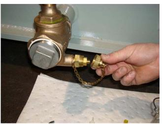
Remove protective cap on sampler cap to expose the fitting.
