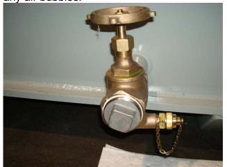
Final inspection of the valve to confirm the valve handle is tight and the area is dry.
