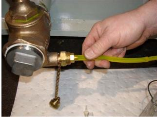
Loosen sampler fitting about two turns prior to installing the hose.
