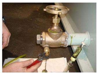
Close drain valve handle (clockwise). Close sampler fitting into the closed position tighten with wrench and remove hose.
