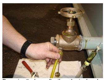
Removing the hose after the valve is closed.
