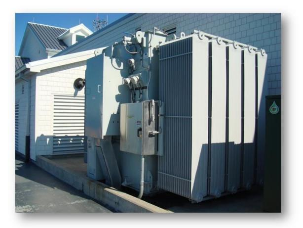
Note that the above transformer although outdoors, is installed directly against the building wall. The transformer HV is 25 kV class, is filled with fluid classified as "less-flammable" and is "curbed" for fluid containment as required for both the FM Approval and UL Combination Classification/Listing.
