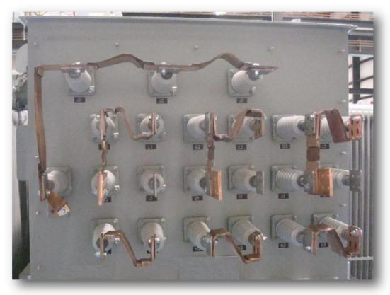
The nameplate details the placement of all high and low voltage bushings as well as the termination requirements for each configuration. Due to the possibility of making connection errors, it is recomended that after
