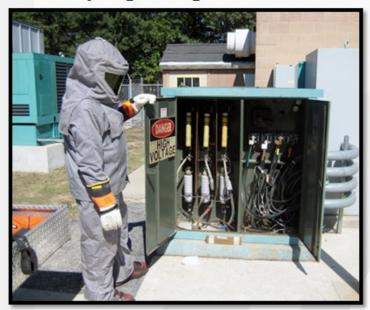
The ability to assess the general condition of the liquid filled transformer through dissolved gas analysis (DGA) represents a significant advantage over dry type transformers. Monitoring the dissolved gas contents over time provides the opportunity to enact preventative measures to minimize the potential of failure.
