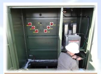
Completing installation of breaker in PCT retrofit transformer
