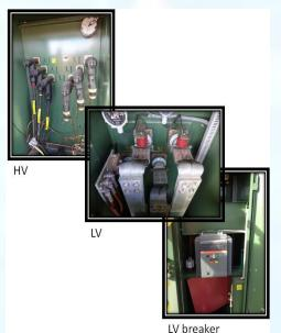
High voltage elbows, arresters, low voltage configurations and terminations, wired accessory packages, and low voltage breakers are but a few of the possible items which may be unique to the transformers supplied for the project.
