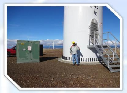
Step-up transformer installed at base of turbine tower
