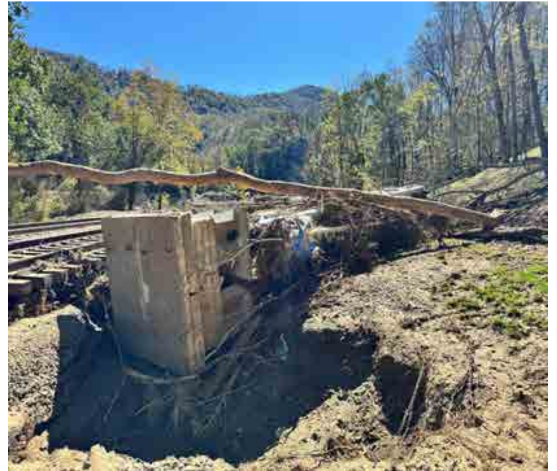
Southbound Signal Cantilever, MP Z-161.02, Green Mountain, NC Washed Out/Destroyed
