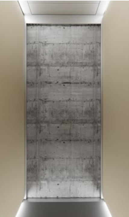
BEFORE WITH EXPOSED MASONRY WORK
