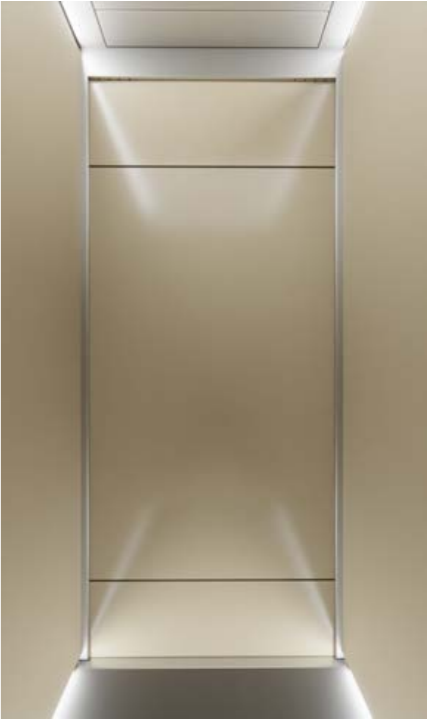
AFTER WITH SHAFT PANNELING BETWEEN FLOORS
