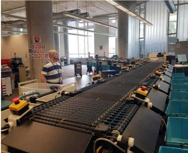
totalAMH systems can work with a mix of various containers depending on the library's desired sorting strategies.
