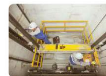
Elevator installation and installation services
