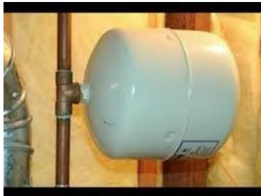
A standard tank water heater can stress your plumbing pipes by the normal thermal expansion that happens during the heating process. A safety device known as a *water heater expansion tank* (sometimes called a *thermal expansion tank*) can help minimize the risk of pressure damage to the plumbing system. (This is normally not a problem on modern on-demand, tankless water heaters--only tank-style heaters are subject to this problem.)
