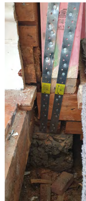
Stud to Beam Connection
