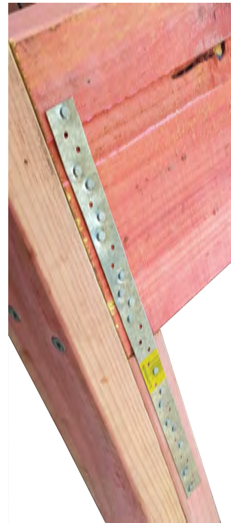
Stud to Beam Connection
