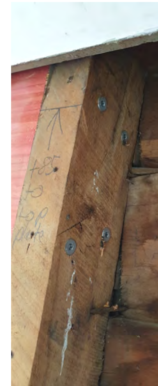
Stud to Beam Connection
