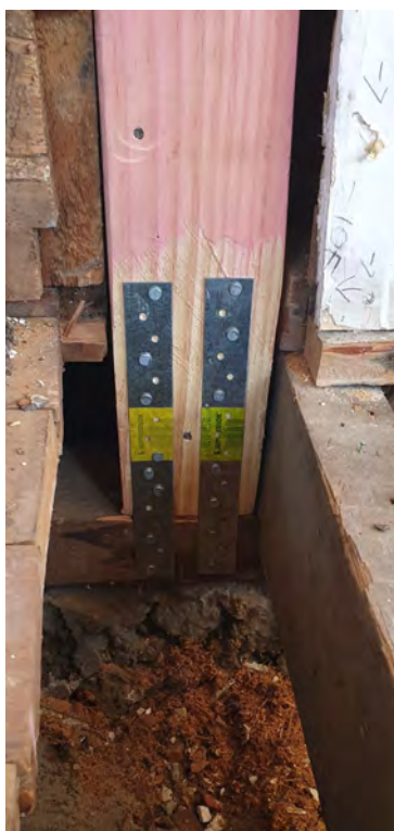
Stud to Beam Connection
