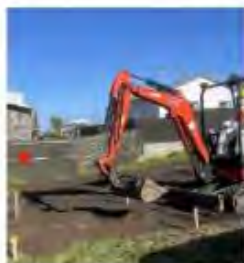
Imported Top Soil being blended with contaminated soil in a 2m square radius around site location SP5 as per CSMP and RAP
