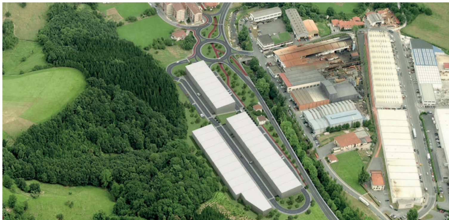
Development of the Kanpandegi industrial estate in Lazkao (Gipuzkoa)
