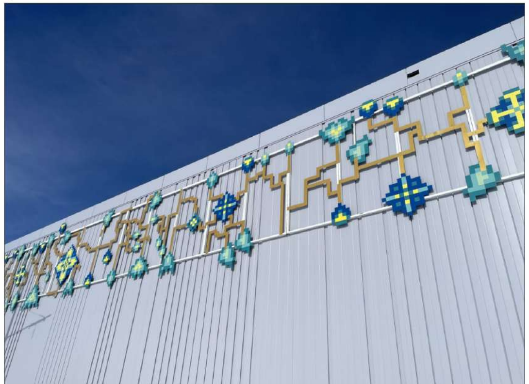
The new artwork In Community We Grow by Shaheer Zazai at the Gerry Wright Operations and Maintenance Facility
