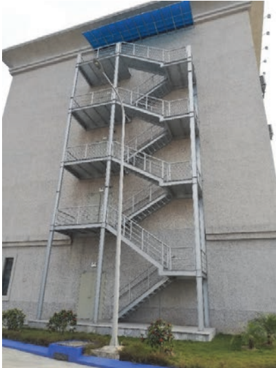
External metal staircase provides a smoke free fire escape path Ever Sun, Vietnam. 2023
