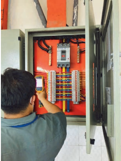
Checking for heat in electrical circuits.. Pung Kook Vietnam 2023
