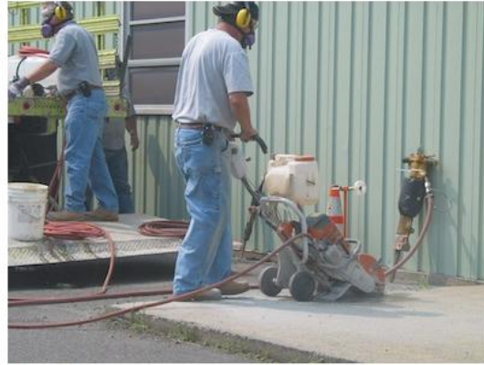
Walk-Behind Concrete Saw with Water Control
