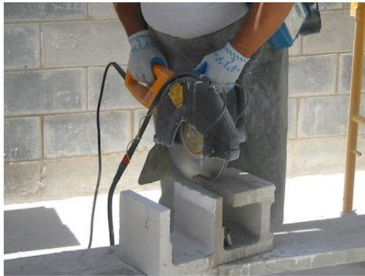
Hand-Held Saw with Water Control
