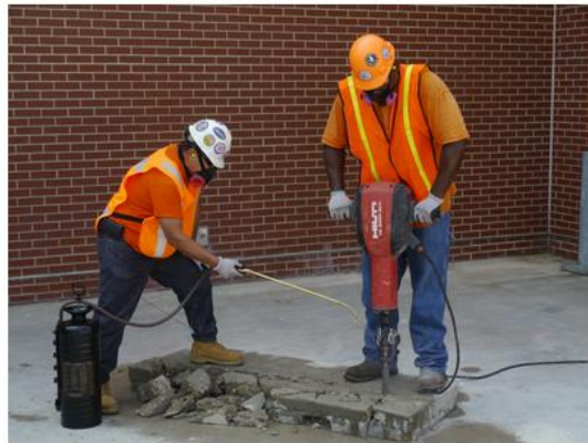
Jackhammer with Water Control
