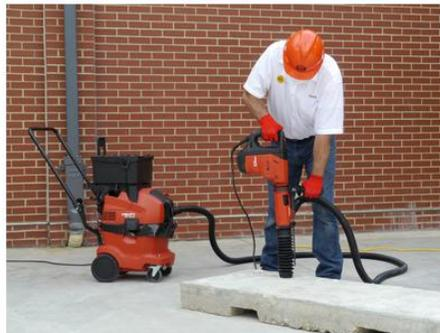
*Handheld Powered Chipping Tool with Vacuum Control*
