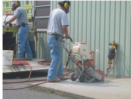
*Walk-Behind Concrete Saw with Water Control*
