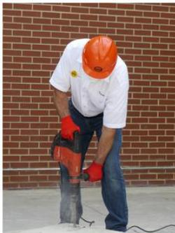
*Handheld Powered Chipping Tool without Control*
